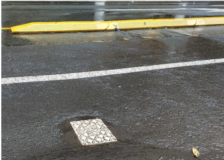
Figure 3 – water pooling in uneven surface
