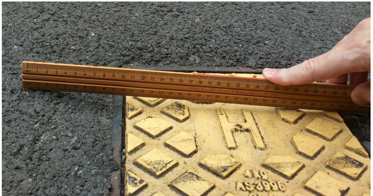
Figure 2 – fire hydrant cap uneven with road surface
