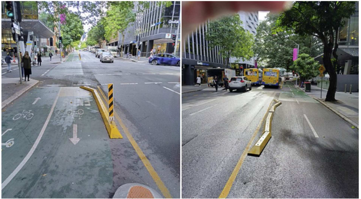
Figure 1 – dislodged dividers
